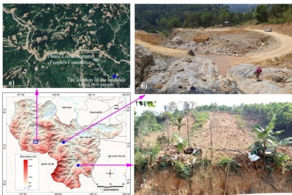
Figure 3. Some pictures of typical landslides: a) A landslide region in Phuoc Loc commune, Phuoc Son district (Google Earth image in October 2021); b) The landslide occurred in Tra Leng commune, Nam Tra My district; and c) The landslide occurred in Tra Van commune, Nam Tra My district. Photographs were taken in April 2021 by Tran Anh Tuan.
